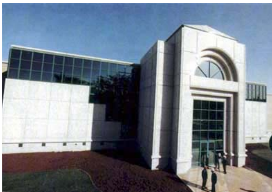
Following 15 years of research, planning, design, and construction, Cincinnati's $ 60 million GAC facility will bring considerable health and environmental benefits to area residents
