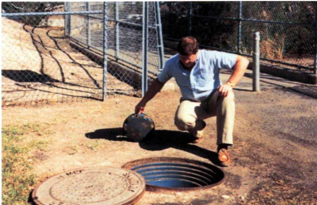
The author holds a carbon canister as he inspects a Sweet Street installation.
