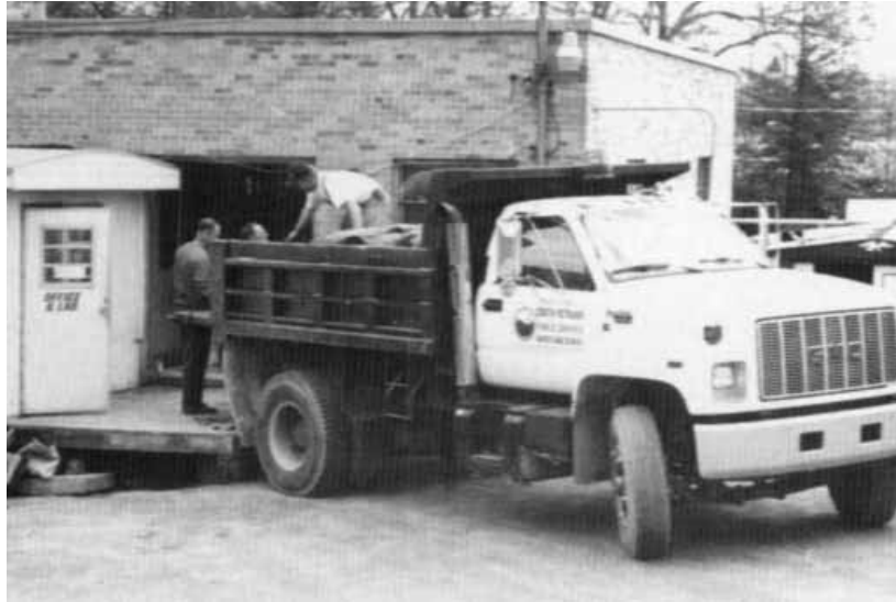
A crew unloading granular activated carbon from South Putnam PSD.
