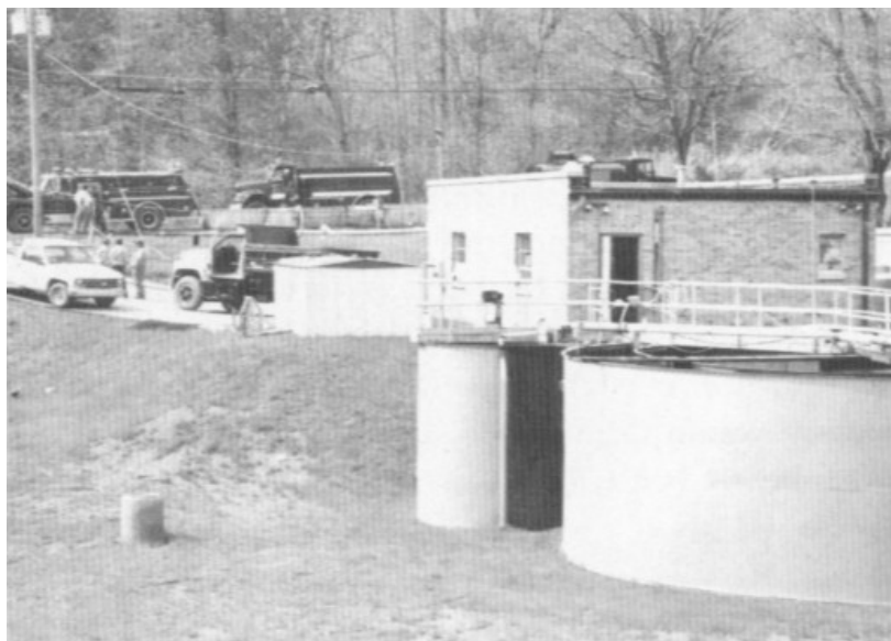
Summersville Water Treatment Plant during the emergency water hauling operation.
