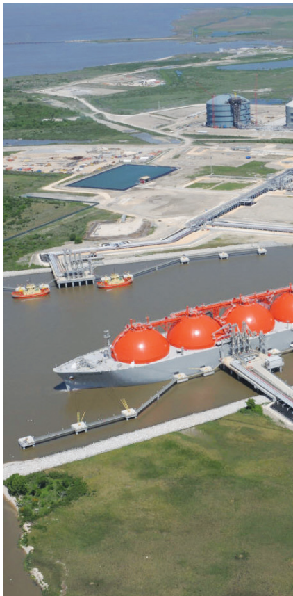
LNG Liquefaction and Export Facility
